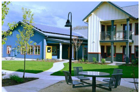
(Willakenzie Crossing with Photovoltaic Panels)
